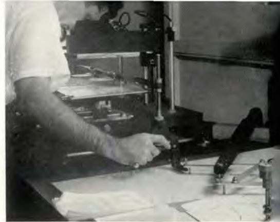
Pantograph is used to trace details and elevations onto charts from aerial photographs.
